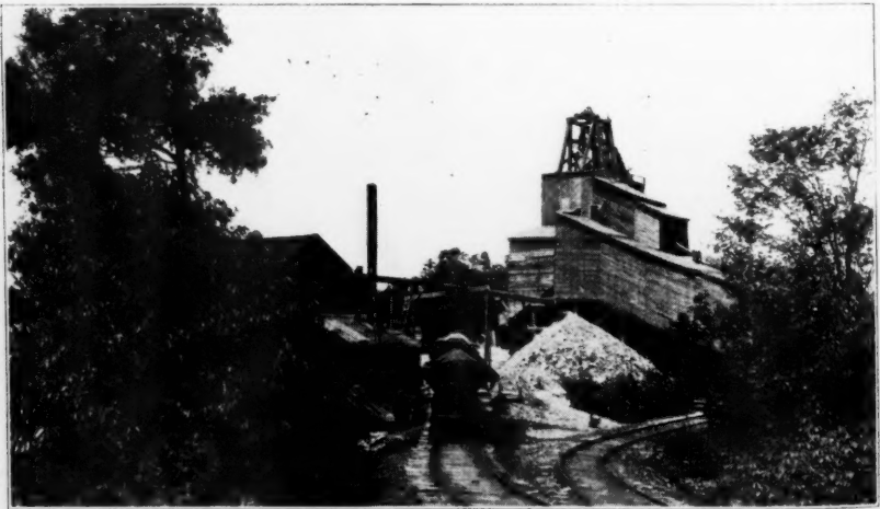
Tracks to Right Lead to Dry Bins While Tracks to Left Lead to Wet Bins.
